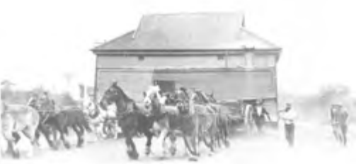
The Bank of Adelaide at Karoonda being shifted by horse teams to make room for a new building to be erected on the site, 1922, State Library of South Australia
